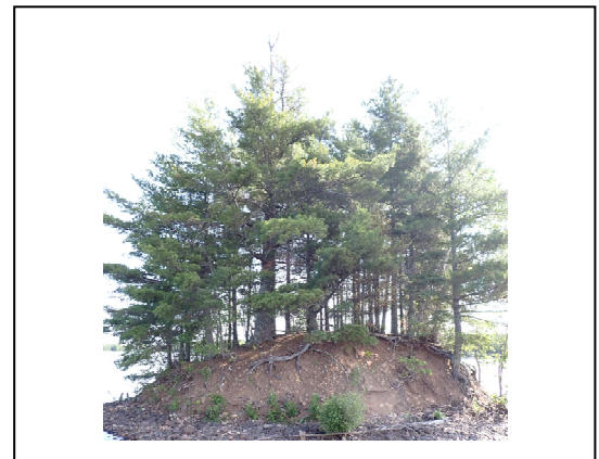
40. Island #8 – Bank erosion
