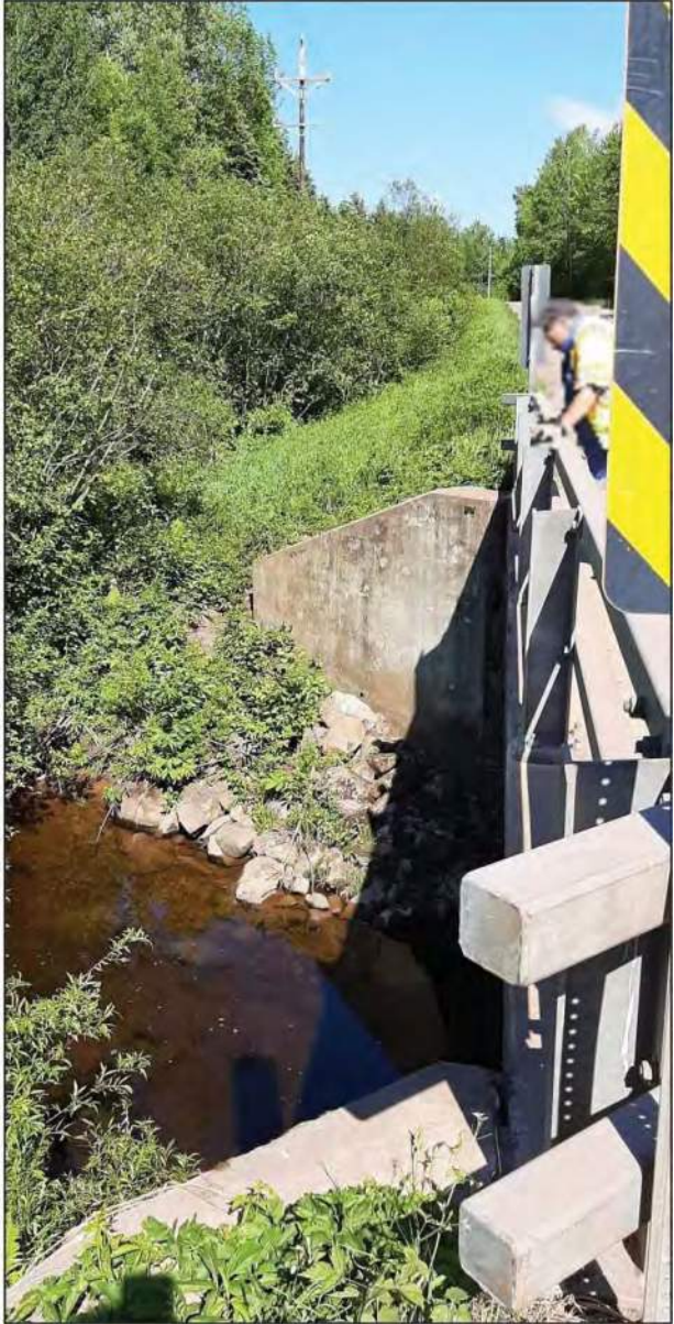
Boomer Creek Downstream from Bridge Photo 9
