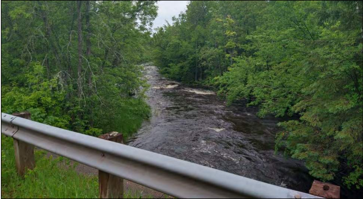
End of Reach 2 – Upstream of Center Drive bridge at 600 cfs
