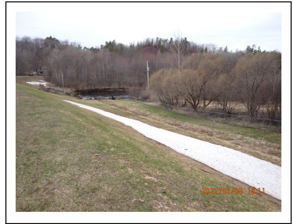
44. Gile Dam Canoe Portage – Downstream side of dam, facing west
