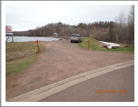
49. Gile Dam Canoe Portage – Entrance to dike walkway
