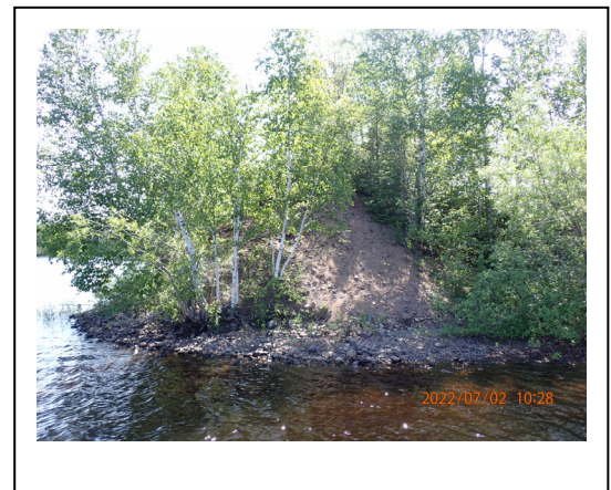
42. Island #9 - Bank erosion
