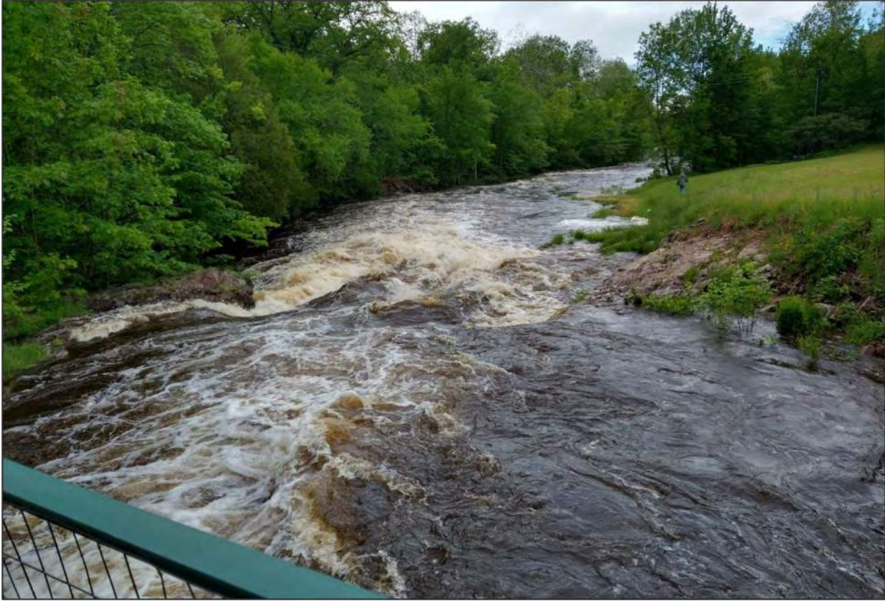
End of Reach 3 – Downstream of Kimball Town Park bridge over Kimball Falls at 1,200 cfs
