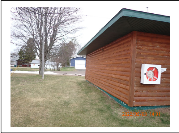
21. Gile Park – Restrooms (2)
