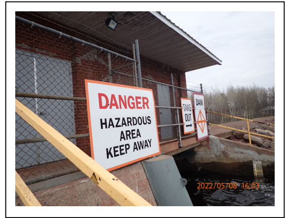
38. Gile Dam Canoe Portage – Intake signage
