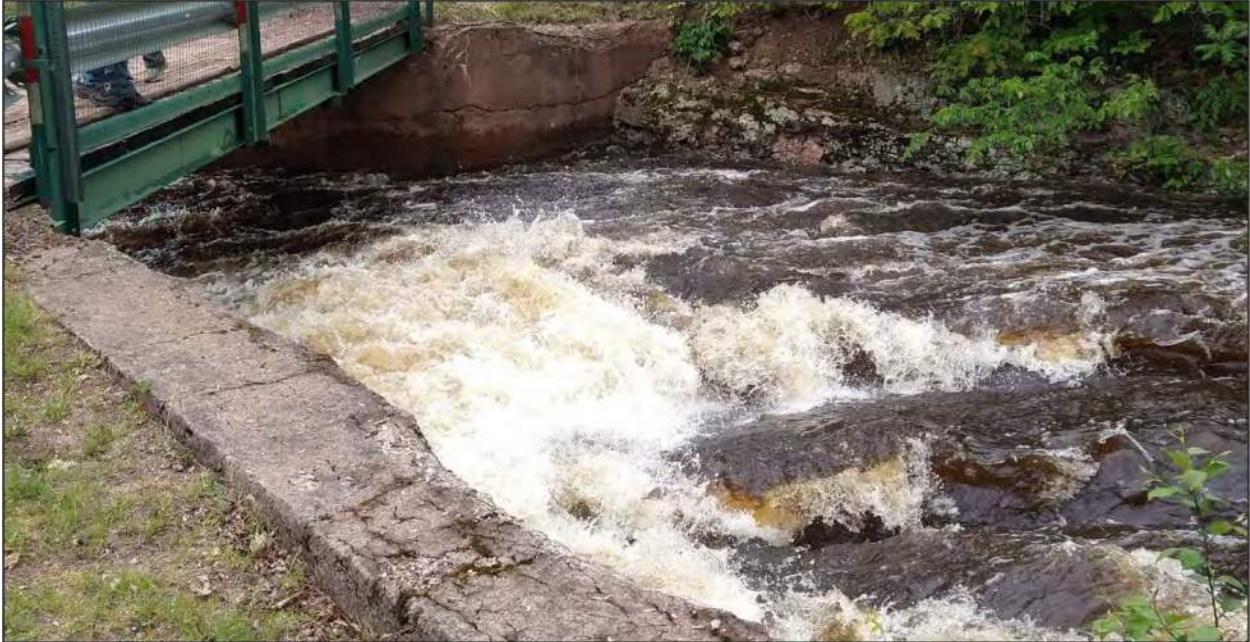
End of Reach 3 – Kimball Town Park bridge upstream of Kimball Falls at 1,200 cfs
