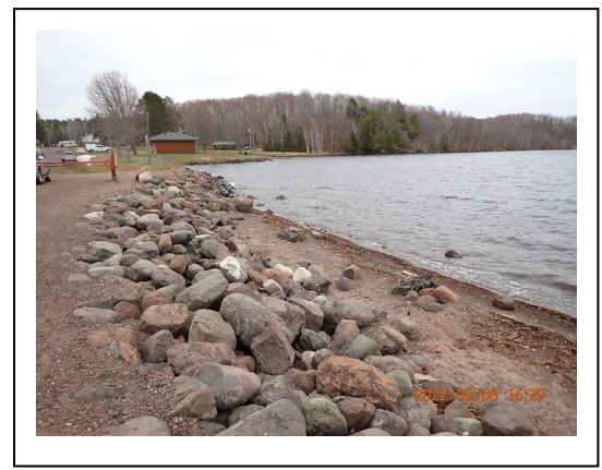
52. Gile Dam Canoe Portage – Riprap and beach, facing east
