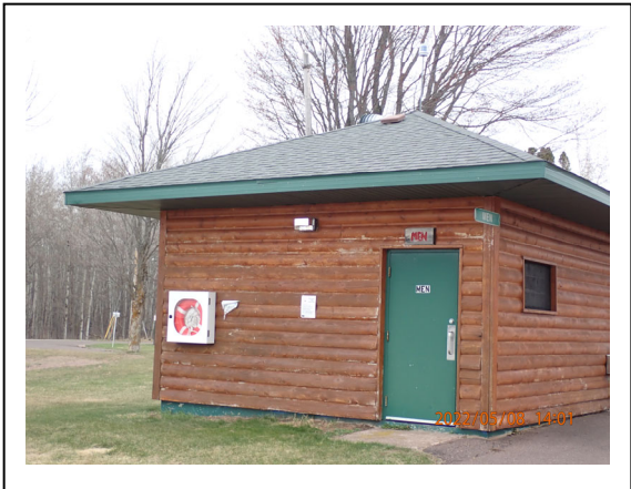
20. Gile Park – Restrooms (1)
