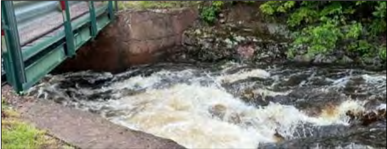
End of Reach 3 – Kimball Town Park bridge over Kimball Falls at 600 cfs
