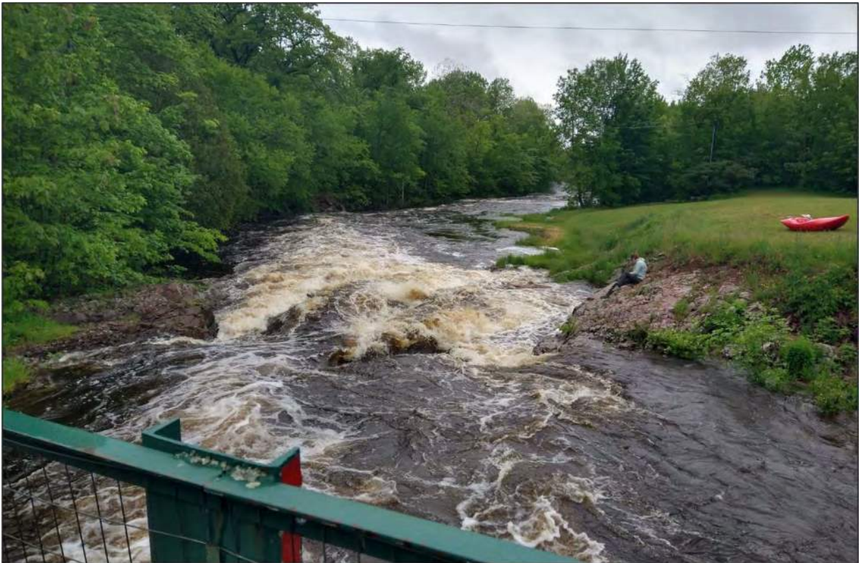
End of Reach 3 – Downstream of Kimball Town Park bridge over Kimball Falls at 600 cfs
