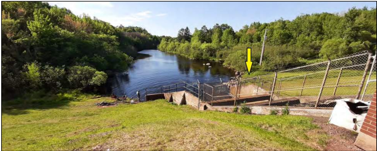
Figure 4.2.2.1-1 Put-In Location and Access at Gile Dam
