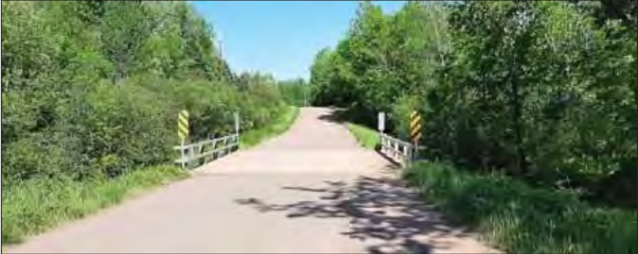
Wall Street Road Bridge over Boomer Creek Photo 7
